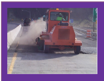
C leaning prior to the placement of the Tack Coat materials
