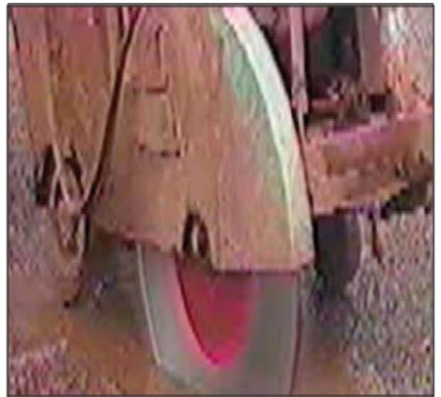
Saw cutting a repair area
