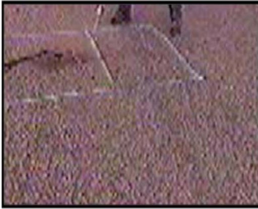
Marking a repair area
