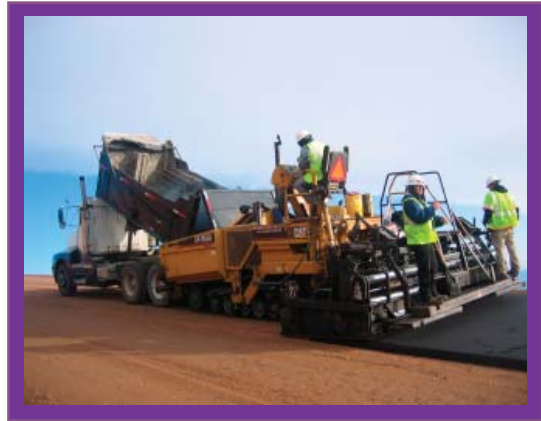
Paving with Superpave HMA
