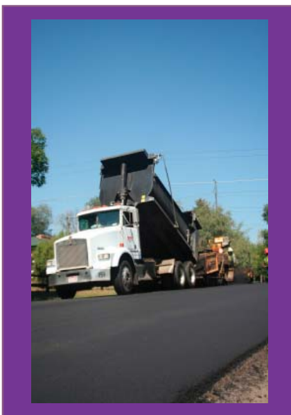
Paving City streets utilizing the "Superpave" Technology
