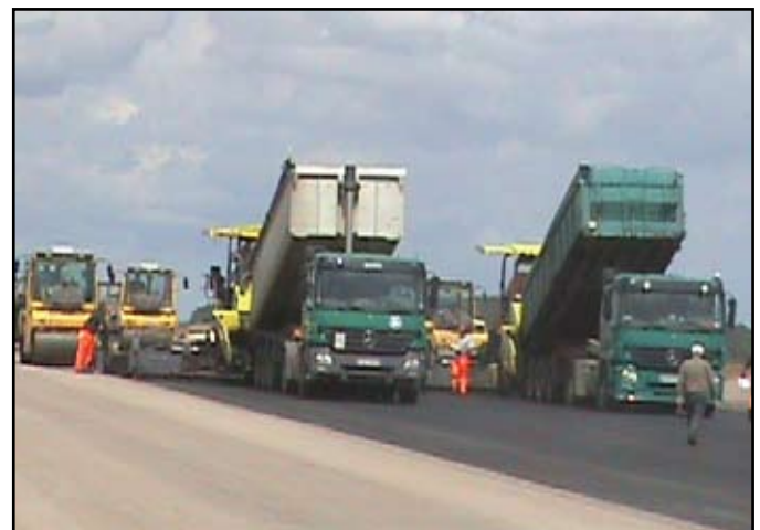
SMA overlay on runway at Spangdahlem Air Force Base, Germany
