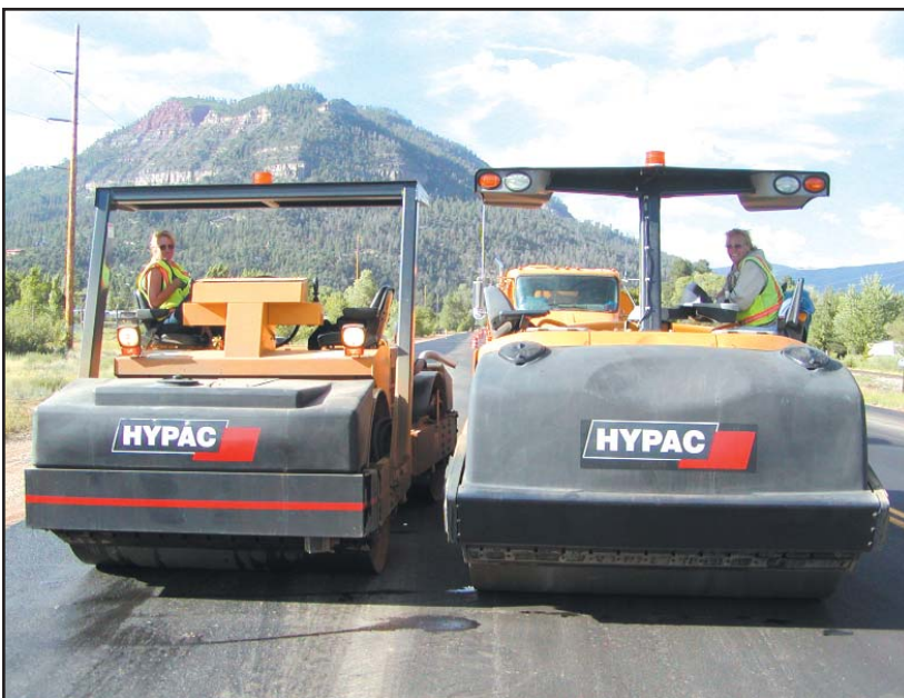
Colorado highway construction, 2004.
