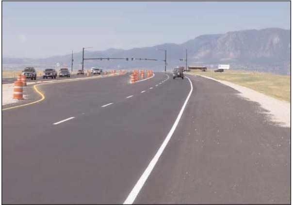
US 24 east of Colorado Springs, widening and asphalt overlay project, Summer, 2004 Contractor: Rocky Mountain Materials and Asphalt, Colorado Springs Agency: CDOT Region 2 Colorado Springs Residency
