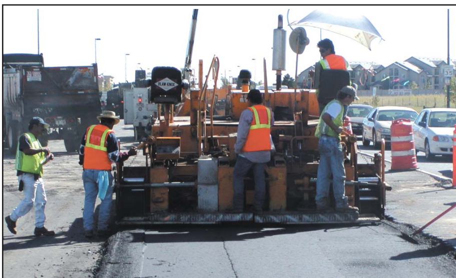
Perpetual Pavement Construction on Tower Avenue in Denver, Colorado. Contractor: Asphalt Specialties Company Inc.
